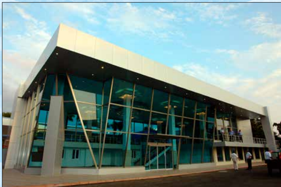
Kobuleti railway station (Georgia)
