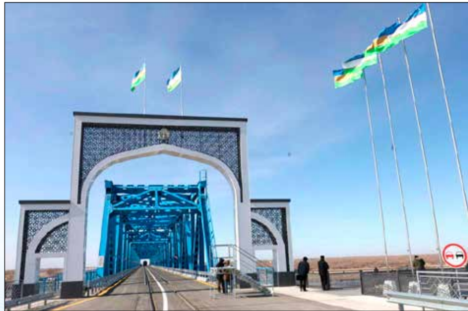
A new combined 423-metre road-and-railway bridge connecting separate districts of the Republic of Karakalpakstan and Khorezm region and an 85-kilometre railway line from the Karauzak district via the Amu Darya and Gurlen districts to the Shavat district
