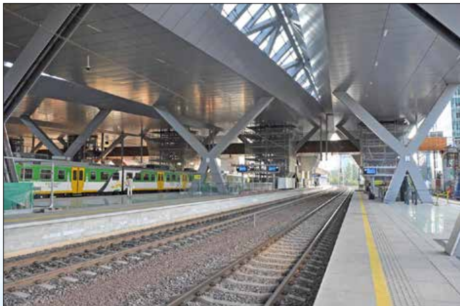
The Warszawa Zachodnia (West) railway station after reconstruction
