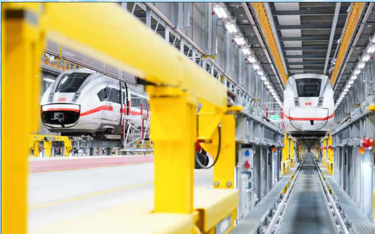
ICE 4 high-speed electric trains undergoing scheduled maintenance at the new centre in Cottbus (photo: DB AG)
