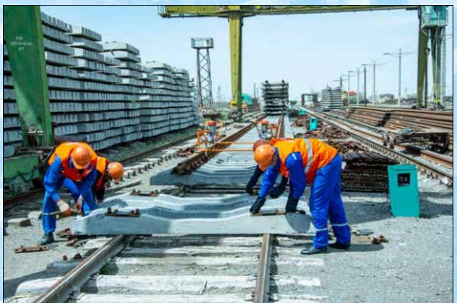
Works for the construction of new railway lines
