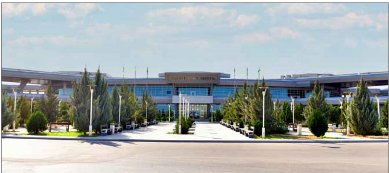
International passenger bus station in Ashgabat
